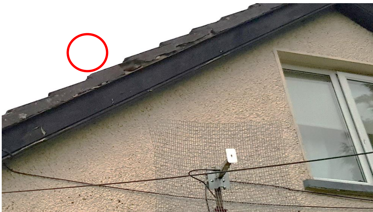
Figure 4-13: Gaps in mortar
